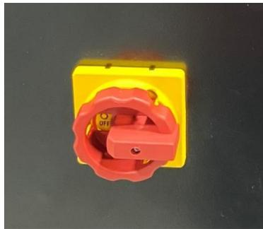
Figure 1: Main shut off switch with Lock Out Tag Out (LOTO)
